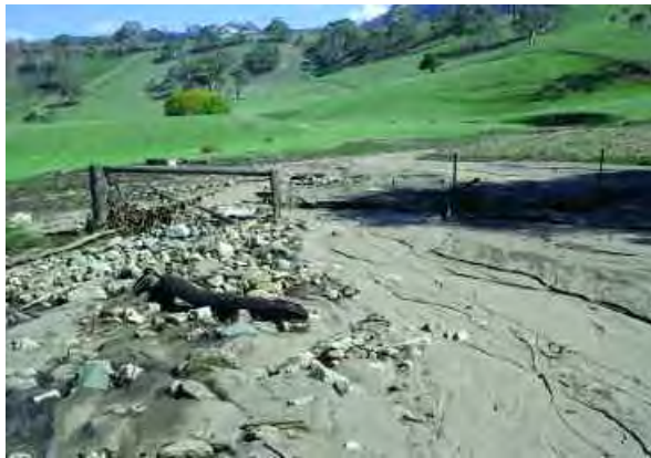
Severe sediment deposit at Frenchman's Creek, Omeo.
