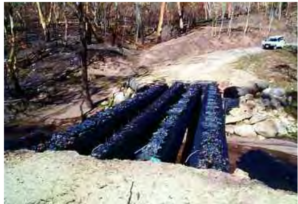
One of the bridges in State forest that needed replacing after the fires.
