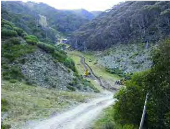
Construction of the new 1.4 km water supply line at Mount Hotham.
