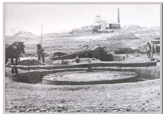
Photo: A horse-driven puddling machine in Central Victoria in the 1880s (DEPI)
