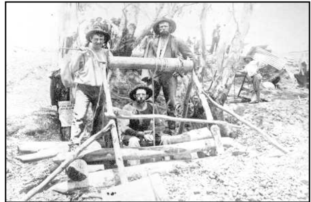
Photo: Members of the Lockett and Scholes family of Waanyarra at a shaft with a windlass
