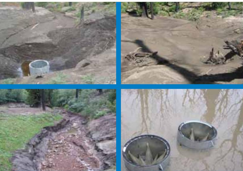
Culvert risers help to slow water down at road crossings, which allows silt to drop out of the water. Once a grass cover is achieved the risers are removed and the stream is able to reset, thus stabilising the soil. This photo shows a culvert riser operating during a high rainfall event, New Years Eve, 2009.
